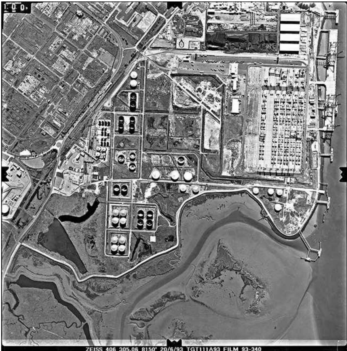
UPSTREAM END OF SITE SHOWING BP OIL TERMINAL
