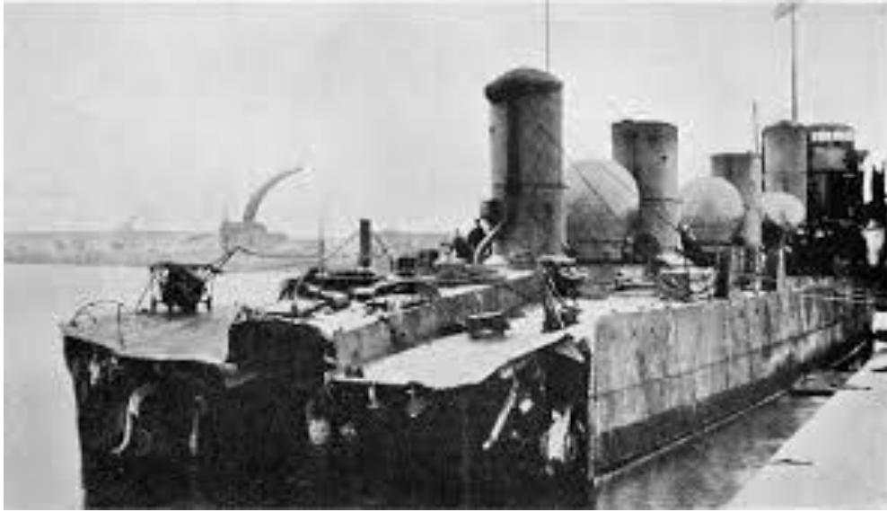
DAMAGE TO ZULU
