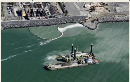
outer, temporary dike at the Fehmarnbelt Tunnel. temporary dike has until now shielded the construction site at the tunnel portal from the water. "But since the entrance to the tunnel portal is now under water and we have completed the 200-meter-wide permanent dike, the outer, temporary dike is no longer needed and can therefore be removed." said Femern. Construction of the Tunnel
