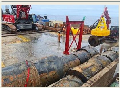
Koole Contractors from Vijfhuizen has started the actual salvage of the coaster Verity. It arrived with the Jifmar push tug Voe Earl and the pontoon K10031 carrying a 200 tonne Liebherr crane at the point in the German Bight where the Verity sank on October 24 after a collision with the bulk carrier Polesie. In the meantime, after the hatches had been lifted, the first rolls of strip steel with electromagnets have been removed from the ship. This
