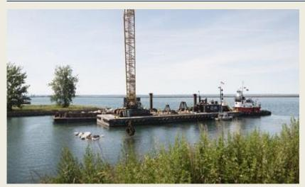
Armor stone is being installed at Wilkeson Pointe in the former commercial shipping slip, the USACE Buffalo District said. According to USACE, this will create a wall in order for clean, dredged sediment to be placed in the slip. Approx. 285,000 cubic yards of clean sediment collected from the Buffalo River over a six year period is set to be placed in the slip, creating 6.7 acres of coastal wetland habitat.
