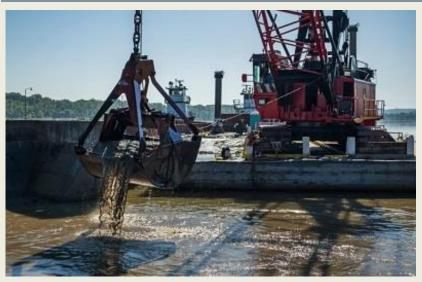
Maintenance work is moving forward at Markland Locks and Dam in Warsaw, Ky, USACE said in its latest project update. Last week, USACE dredging team was onsite dredging inside the 600' lock chamber, near the upstream land approach wall, and in the harbor area near the project site. Navigable channels are dredged throughout the U.S. to keep traffic operating efficiently, said USACE. The
