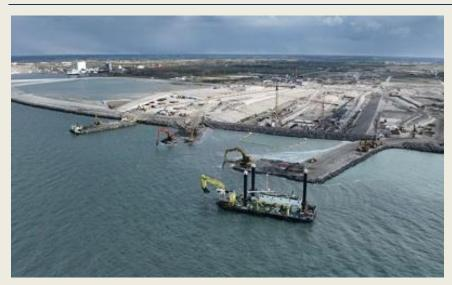
A large part of the outer, temporary dike has been removed at Fehmarnbelt Tunnel, Femern A/S said. Shortly after the tunnel portal was covered by water, Fehmarn Belt Contractors started digging away the outer, temporary dike. The temporary dike has until shielded the construction site at the portal from the tunnel water. "But since
