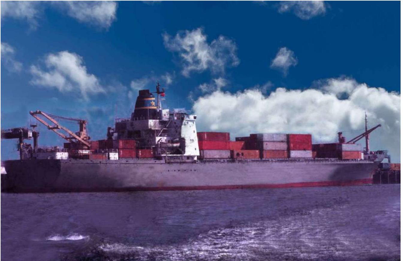
“Antonia Johnson” at Felixstowe in 1982. Built 1971 by Wartsila, Turku, Finland for Rederi A/B Nordstjernan (Johnson Line). Sold in 1985 to Agapanto Holdings (MSC managers) and renamed “Regina D” , renamed “MSC Regina” in 1994 and “MSC Giovanna” in 1998. Broken up at Alang March 1999. (Photo by Tony Wrycraft)
